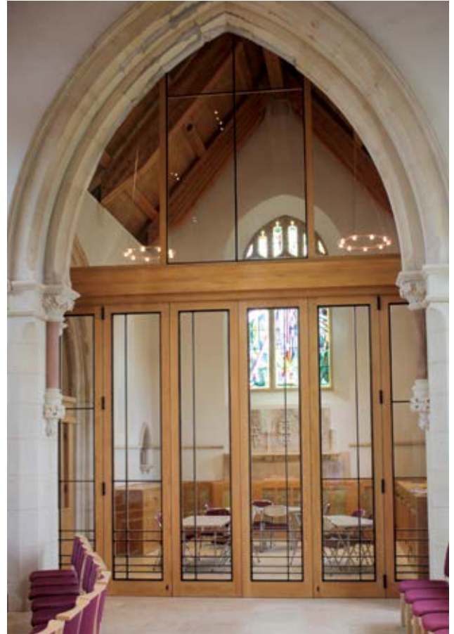
St Nicholas, Radford Semele Caroe & Partners glazed folding door screen and arch above.
