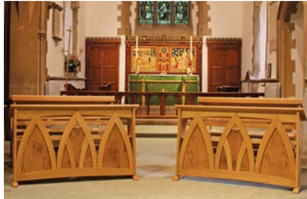
St Mary's, Princes Risborough Choir stalls using arches with feature oak panels to support the readers.
